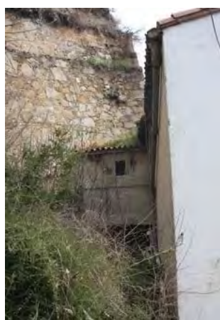
F9 Façana principal oest (Volum C)
