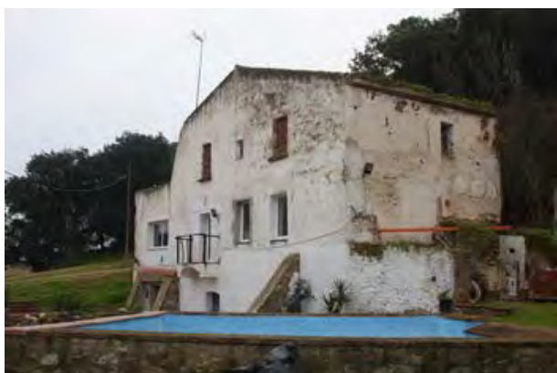
F7 Façana principal i bassa (Volums A i D)
