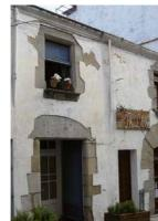
This is a group of two "cases de cos" typical of the small towns in the Maresme region from 16th-18th centuries. There were two parallel walls that held a roof which separated ground floor (working area) and first floor (living area). On the facade the openings enhance for their granite stone frames, an architectural
