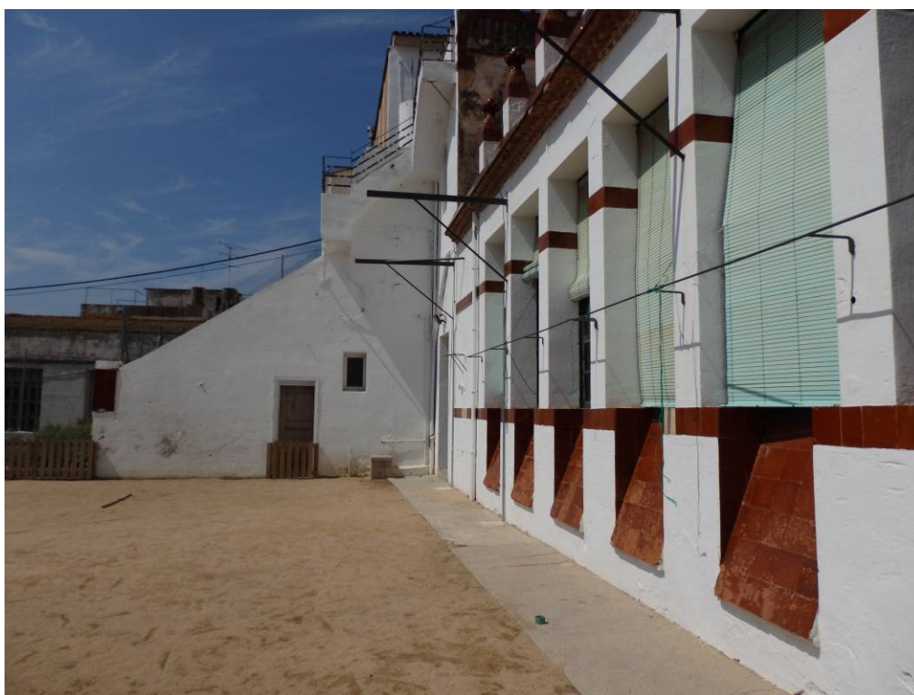
Façana pati interior
